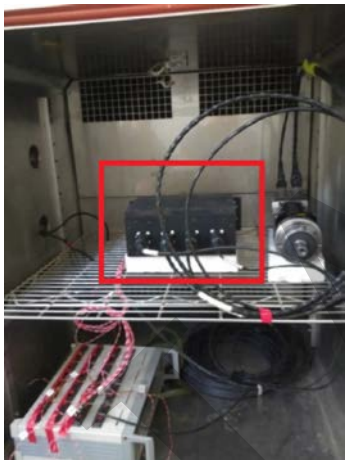
图 9 控制器在环境模拟实验箱内的安置情形 Fig. 9 Installation location of controller in the environmental simulation test chamber
